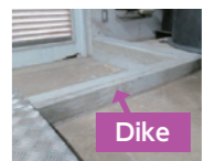
Dike near entrance of the waste water treatment room
