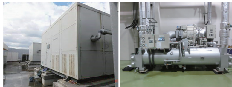
Absorption chiller (gas)
