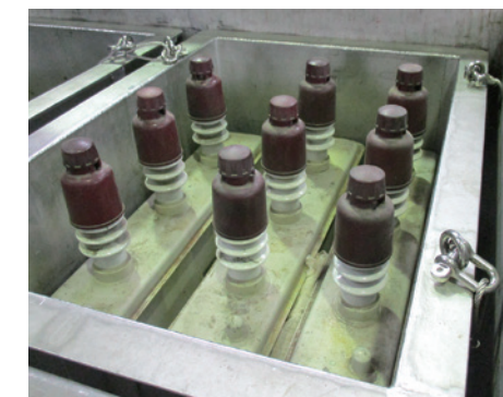
Removal of high-voltage capacitors with highly concentrated PCB
